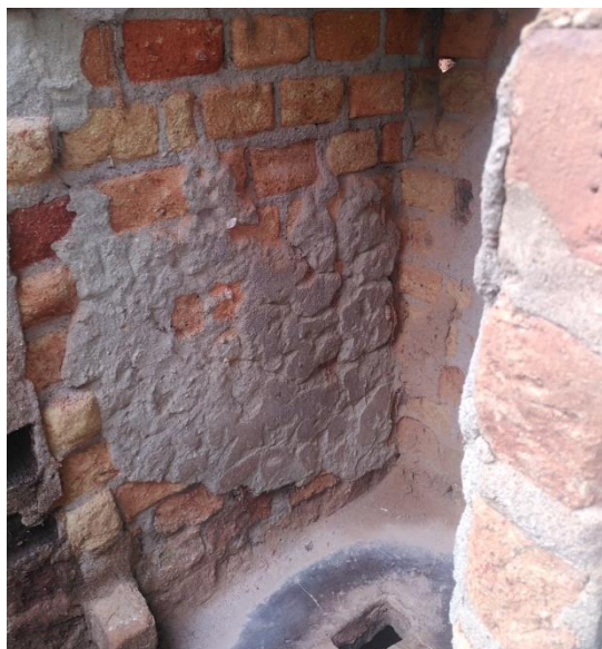
Figure 13: Unfinished pit latrine
